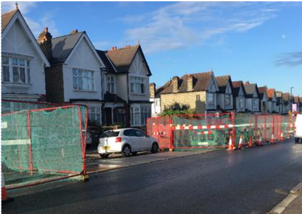
A typical UK Power Network worksite.
