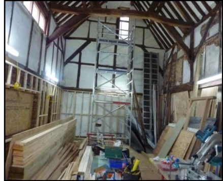
Repairs to the inside of the stable
