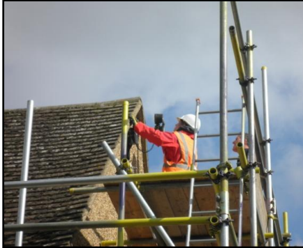
Repairs to the stable roof
